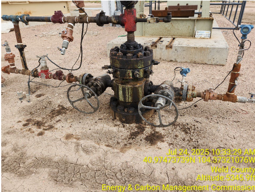
Photo 3 – Stained Soil at 504-2524H Wellhead
