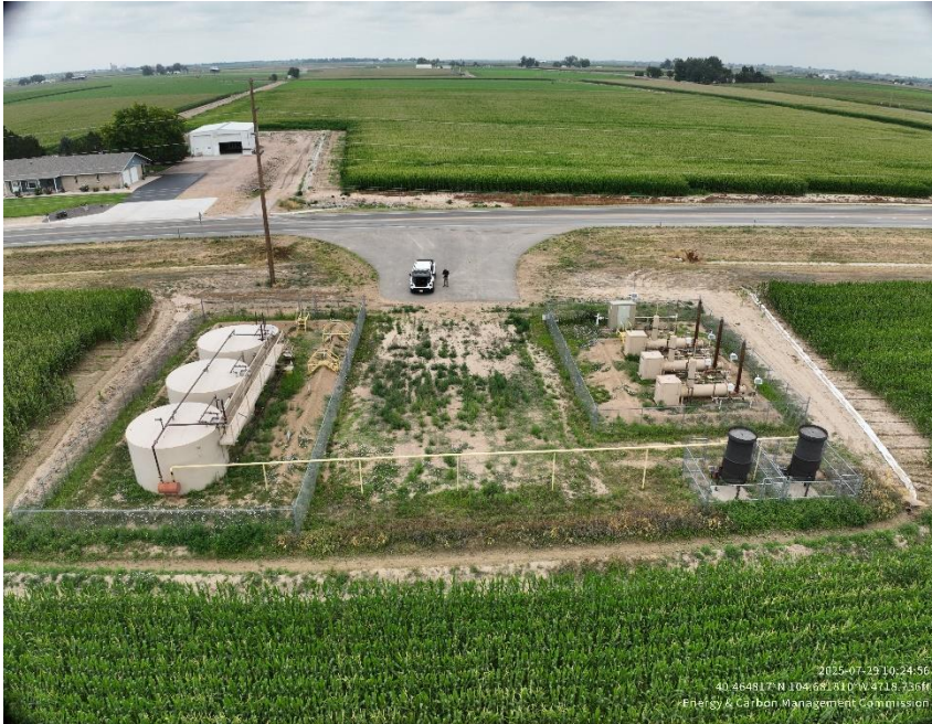
Location and Overgrown Vegetation
