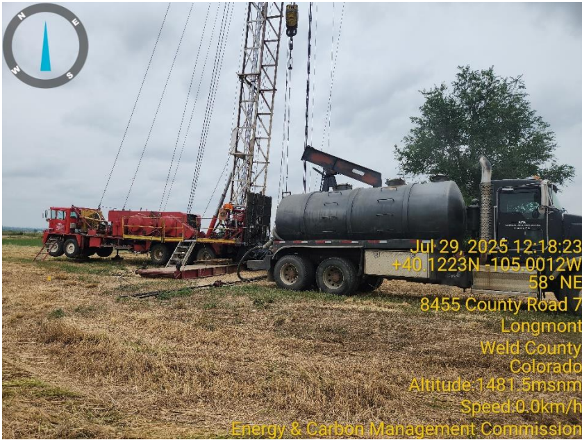
Photo 3 Hot oiler & WO rig.
