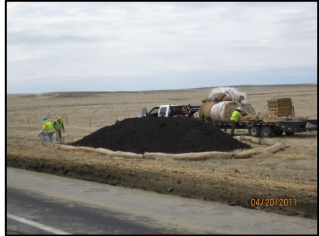
Erosion Logs used for stockpile management practices
