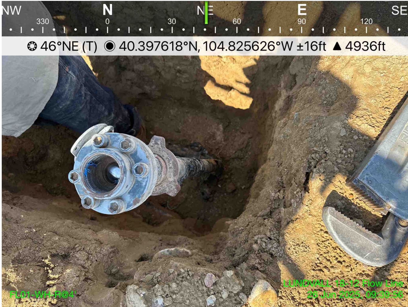
Photo 1: View of flowline wellhead riser, facing northeast
