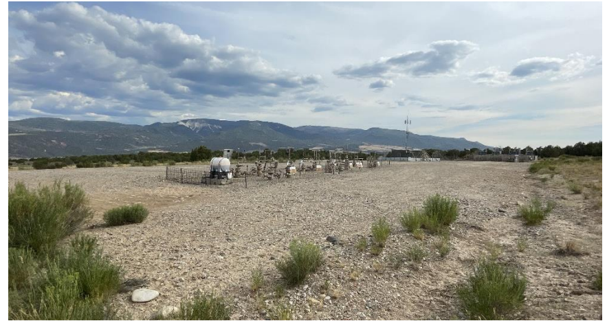
North East corner of location.
