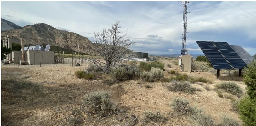
South West corner of location.
