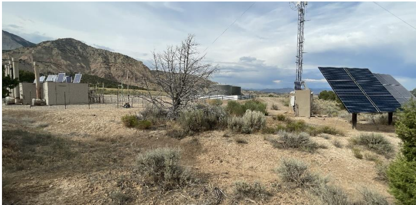
South West corner of location.
