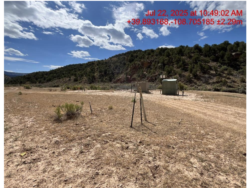
Photo # 0513 NW corner of location
