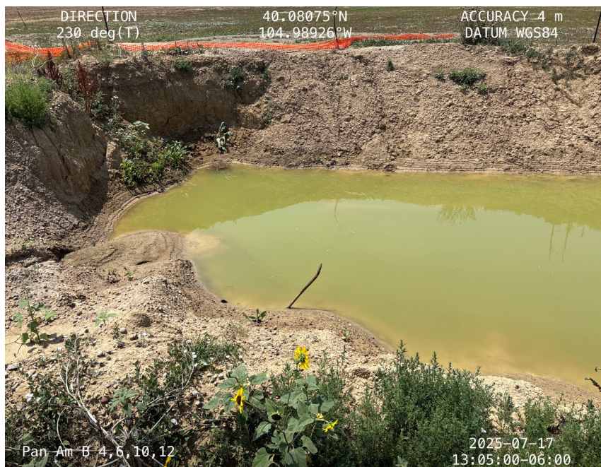
Groundwater within main excavation
