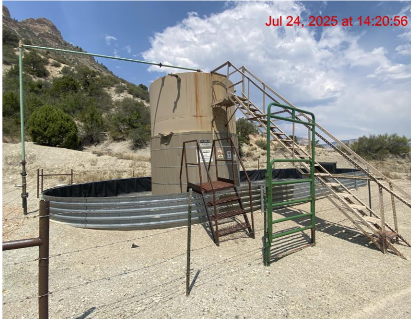
Location/No Battery Sign Posted – Photo #09927
