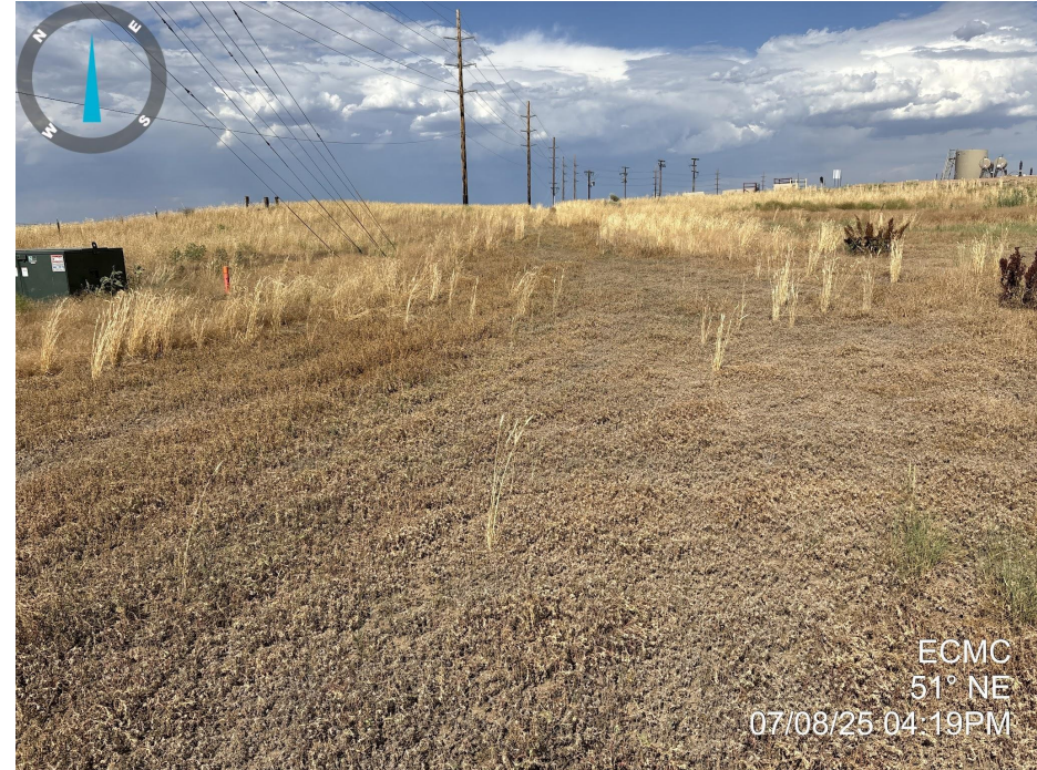
Photo 6. Photo taken of the access road to the well location, facing northeast. See comments under Photo 5.
