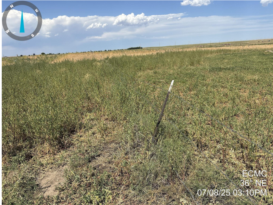
Photo 7. Photo taken of fencing along the access road to the location, facing northeast. Photo illustrates that fencing remains and is in disrepair.
