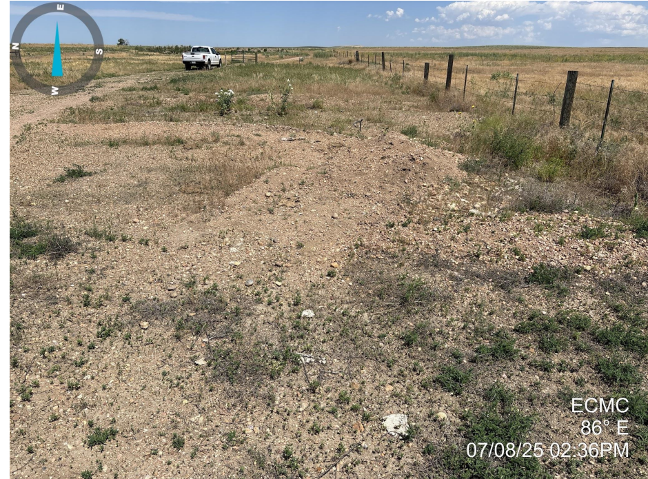
Photo 4. Photo taken of the western portion of the tank battery location, facing east. See comments under Photo 3.
