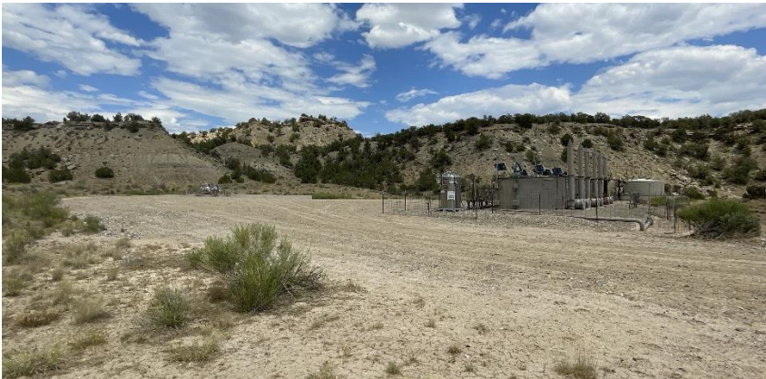
South West corner of location.
