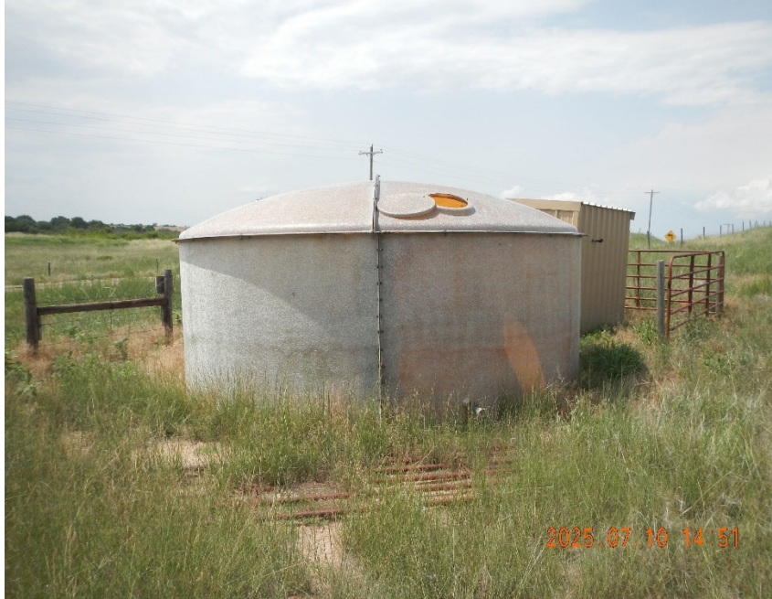
11. Produced water tank located at gathering location.
