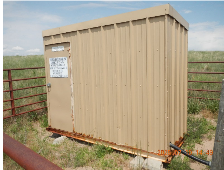
8. View of Separator/Meter Shed.
