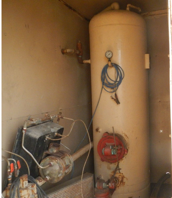
9. Vertical Separator inside shed.
