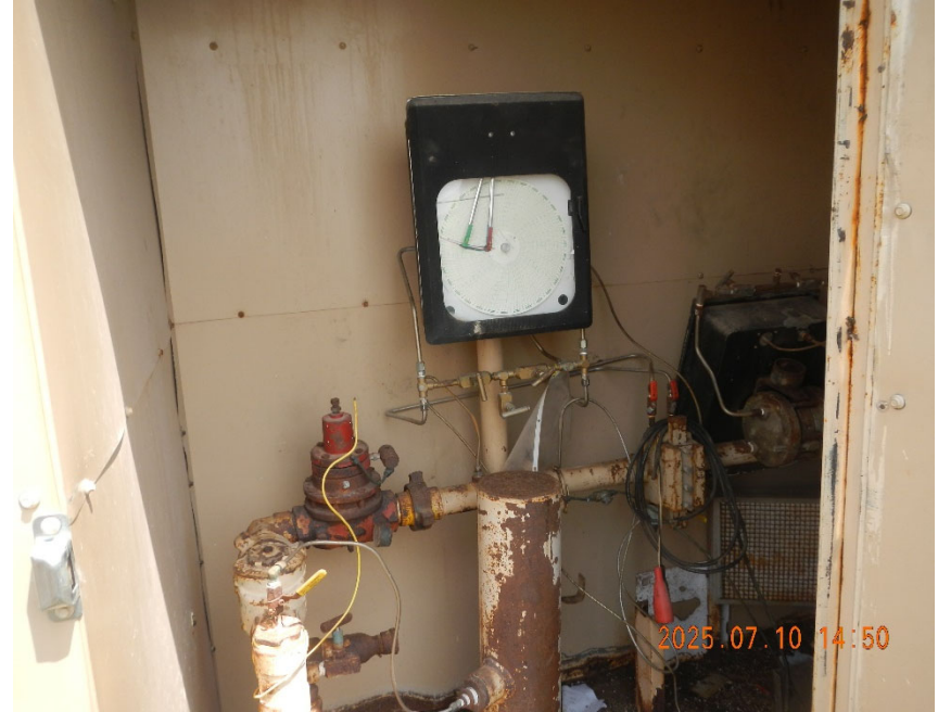
10. Gas meter inside shed.
