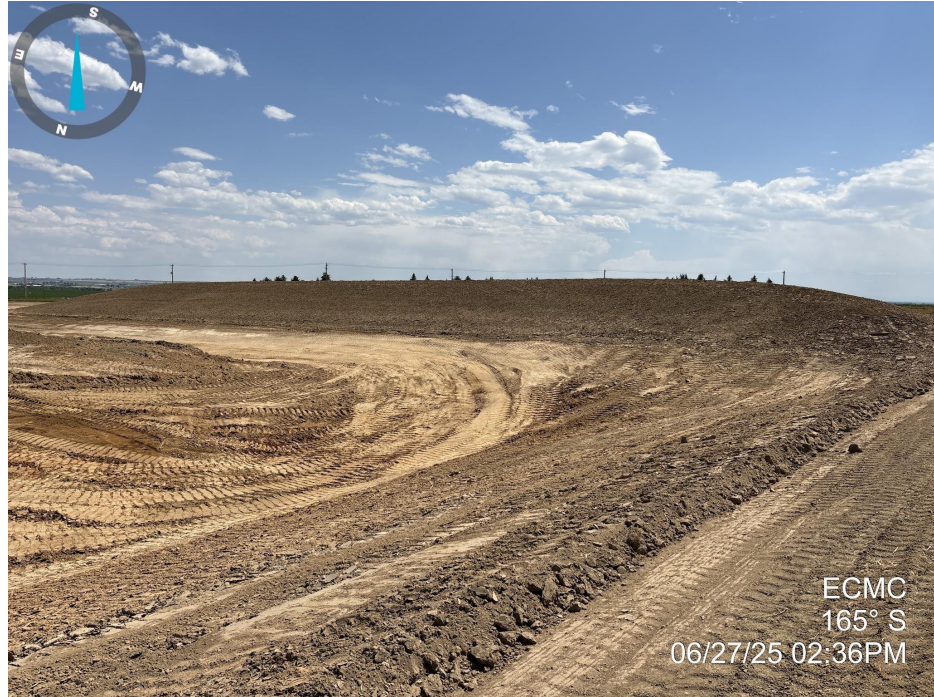
Photo 12. Photo taken of the topsoil stockpile. Photo illustrates the operator has not yet stabilized the stockpile.
