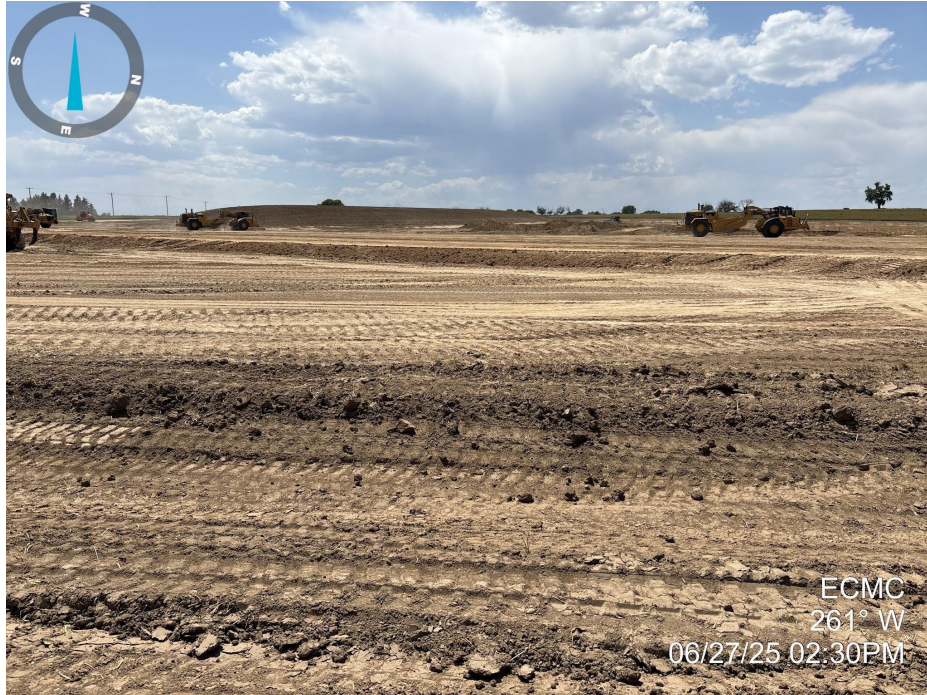
Photo 9. Photo taken from the eastern portion of the location. Photo illustrates the operator is in the process of stabilizing the working pad surface.
