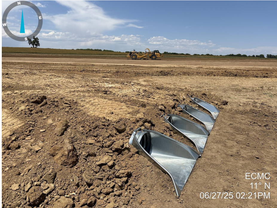
Photo 3. Photo taken from the southern perimeter of the location, facing north. Photo illustrates culverts have been installed near the southwestern entrance to the location.
