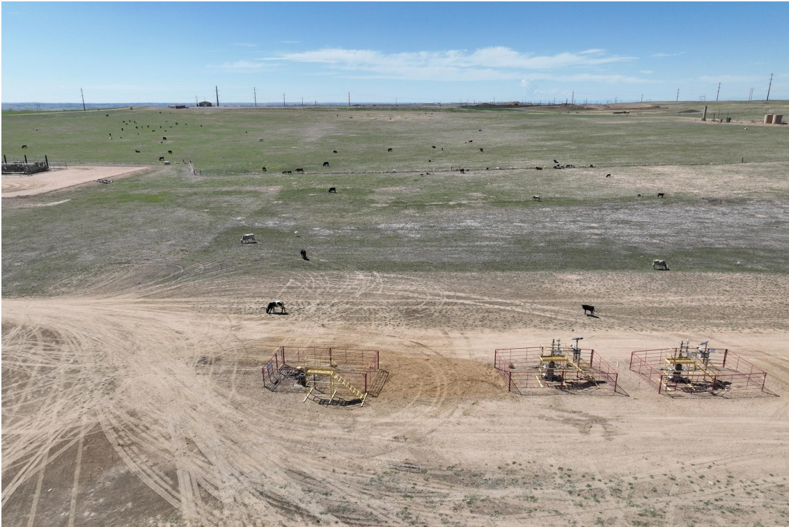
Photograph 3: View facing south as required in Energy and Carbon Management Commission (ECMC) Rule 1004. Photo Taken from GPS 40.130539, -104.738208
