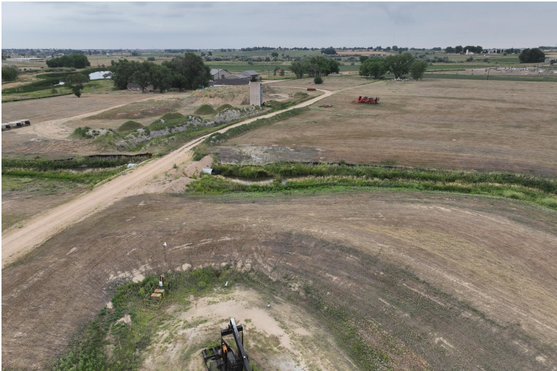
Photograph 2: View facing east as required in Energy and Carbon Management Commission (ECMC) Rule 1004. Photo Taken from GPS 40.122336, -105.016137
