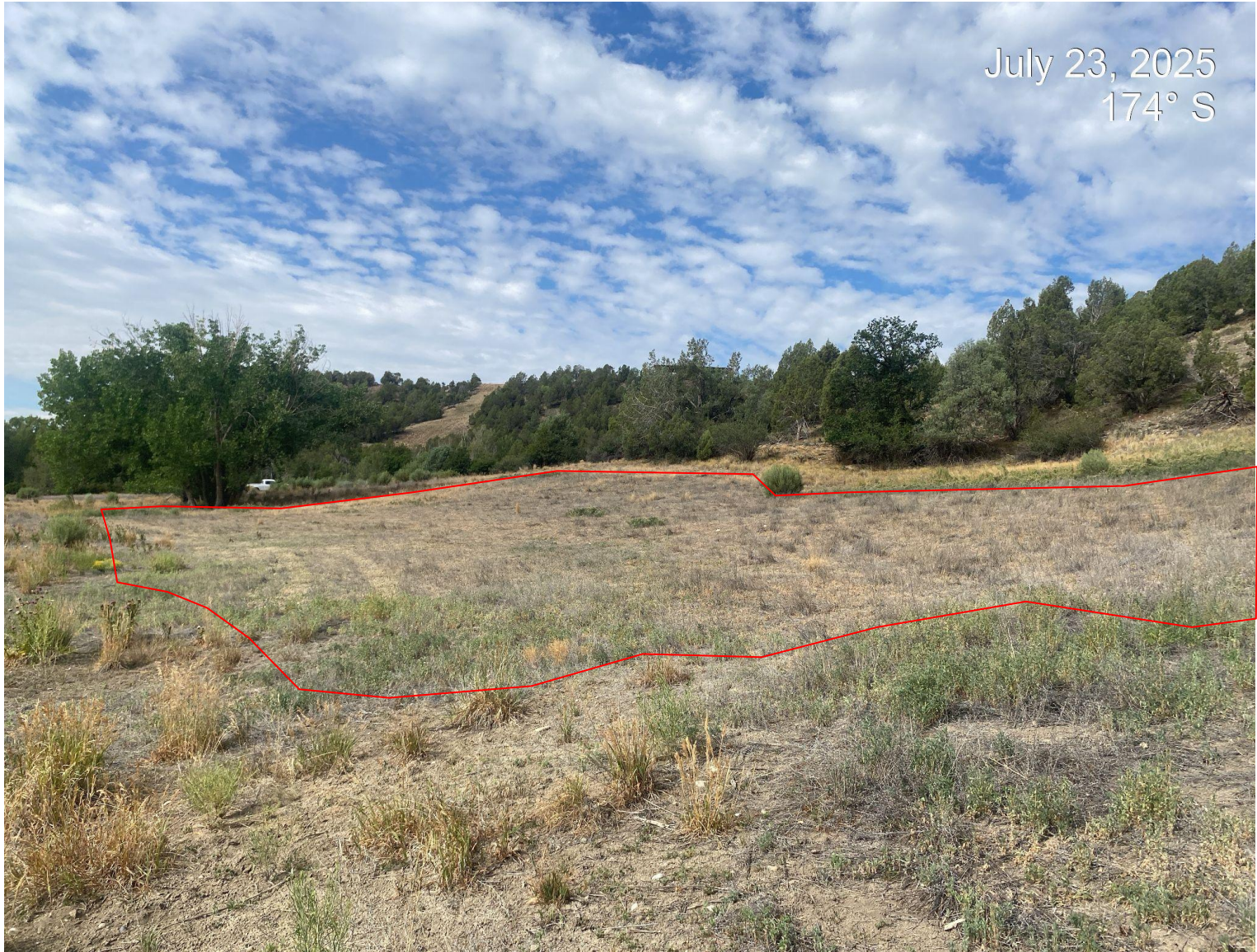
Photo 4. Northwest corner of project area (approximately \frac{1}{3} acre) remains with dense patches of weedy Kochia debris which is interfering with the establishment of desirable species. Additional reclamation work is needed in this area.
