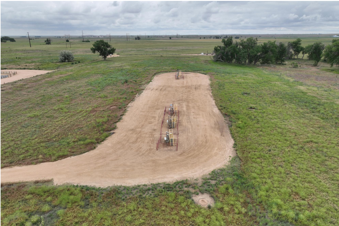
Photograph 2: View facing east as required in Energy and Carbon Management Commission (ECMC) Rule 1004. Photo Taken from GPS 40.158587, -104.638790
