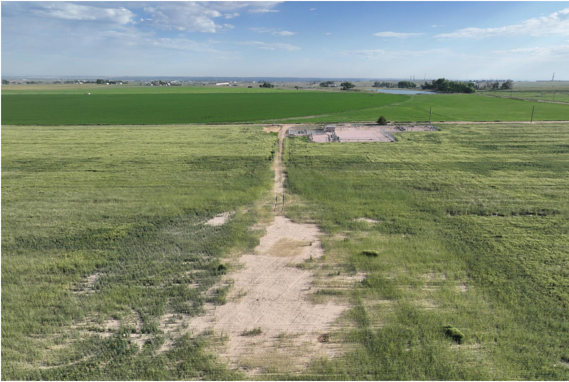
Photograph 1: View facing north as required in Energy and Carbon Management Commission (ECMC) Rule 1004. Photo Taken from GPS 40.229981, -104.756619
