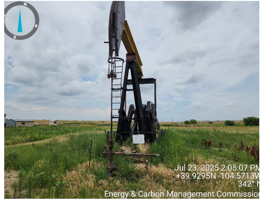
Photo 2 well head and equipment
