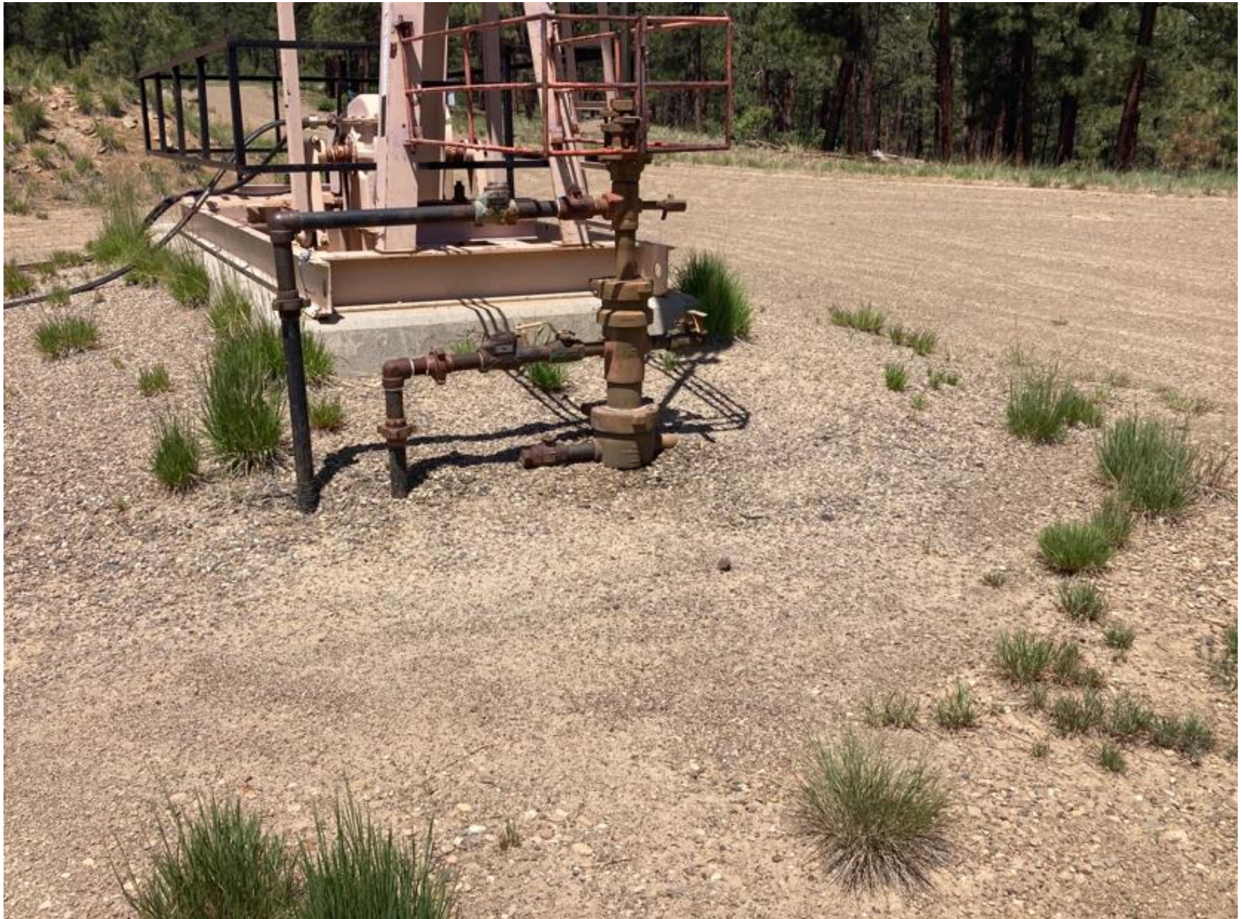
PHOTO 1: THE PACKING HAS BEEN TIGHTENED AT THE WELL HEAD AND THE LEAK STOPPED. ALL IMPACTED SOIL HAS BEEN REMOVED FROM LOCATION AND REPLACED WITH FRESH PAD MATERIAL.
