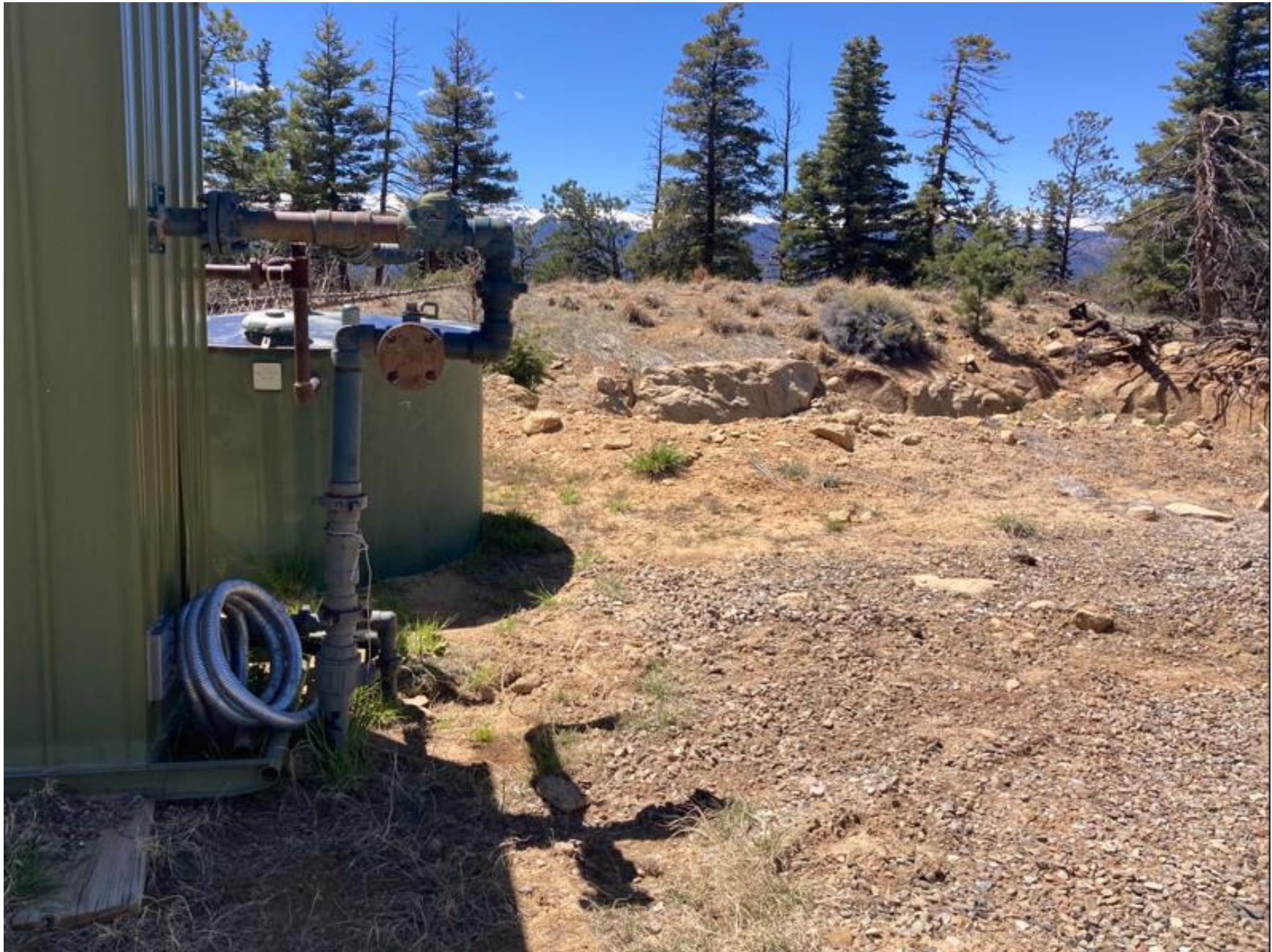
PHOTO 2: THE UNUSED RISERS HAVE BEEN REMOVED FROM LOCATION.
