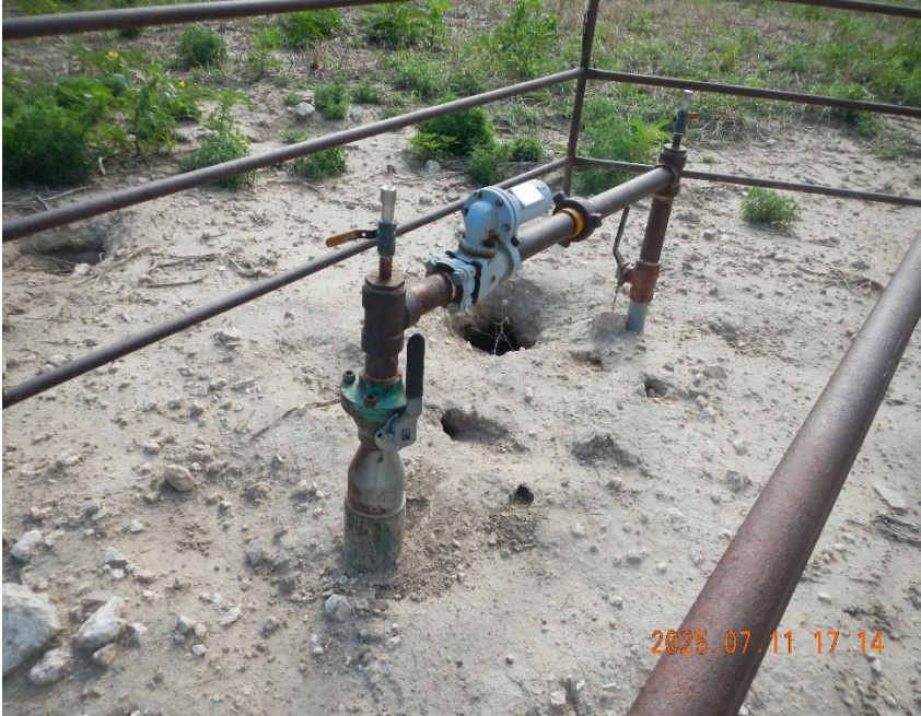
3. View of wellhead. Note no Bradenhead visible at surface.
