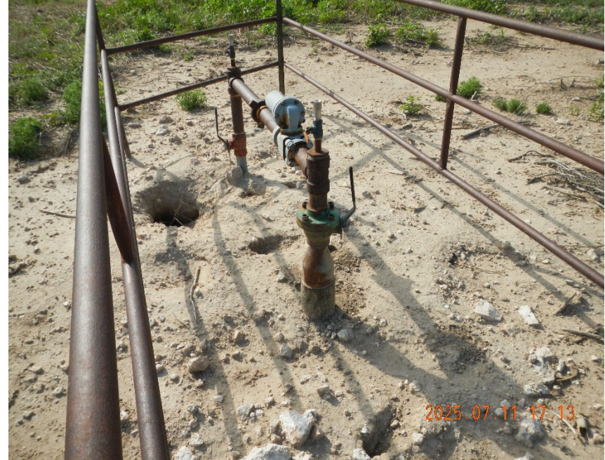
2. View of wellhead. Note no Bradenhead visible at surface.
