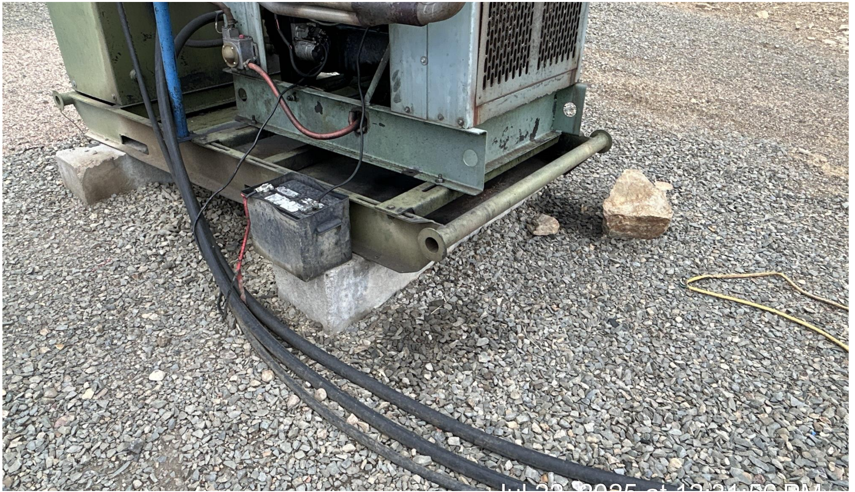
PHOTO 3: IMPACTED SOIL FRONT OF ENGINE SKID
