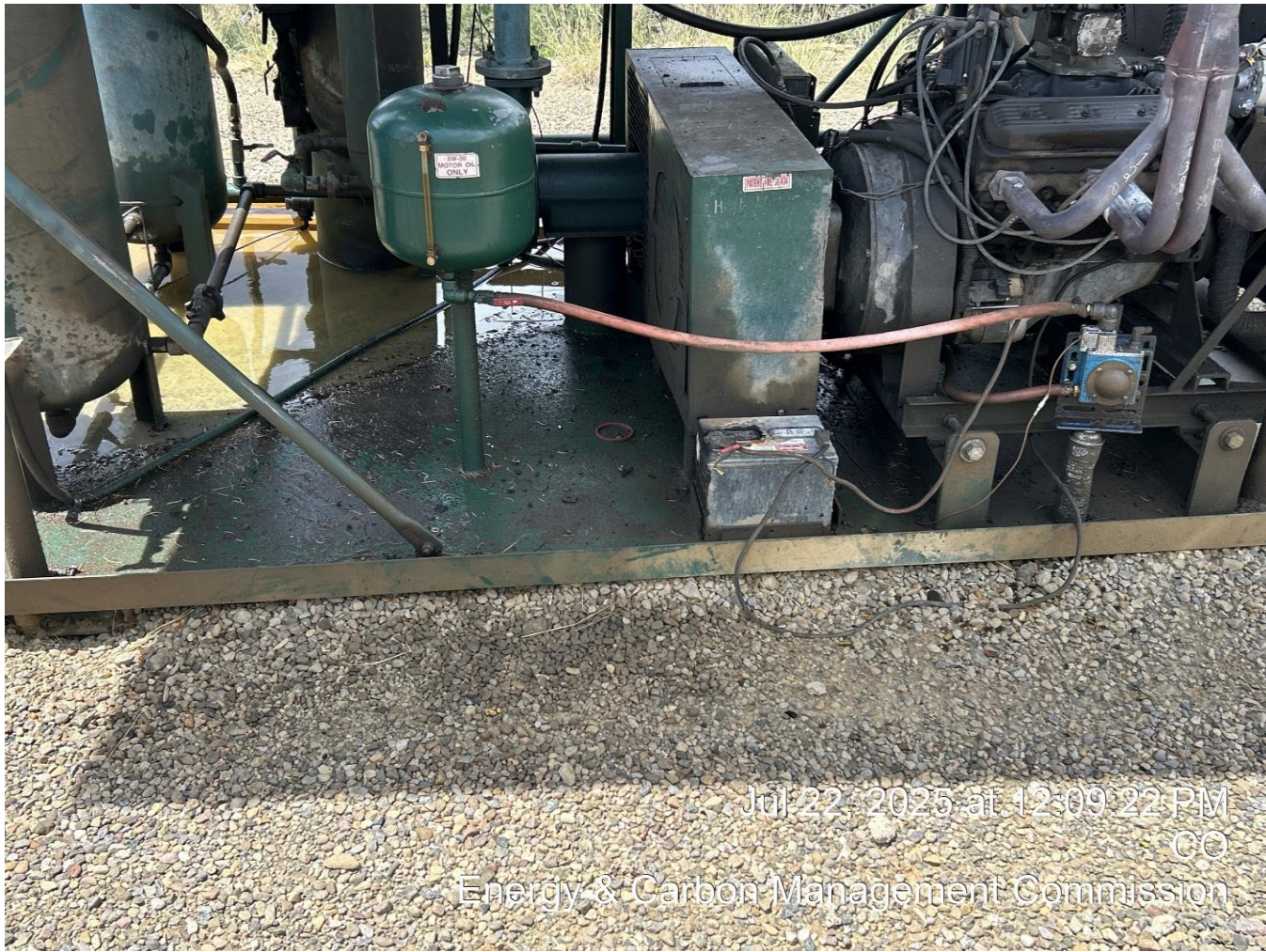
PHOTO 4: Impacted soil at ring
