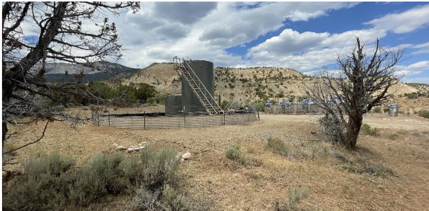
South West corner of location.
