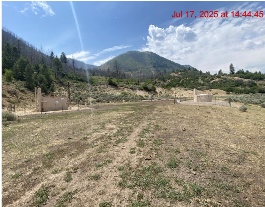
Location Overview/Weeds/Fire Hazard – Photo #09800
