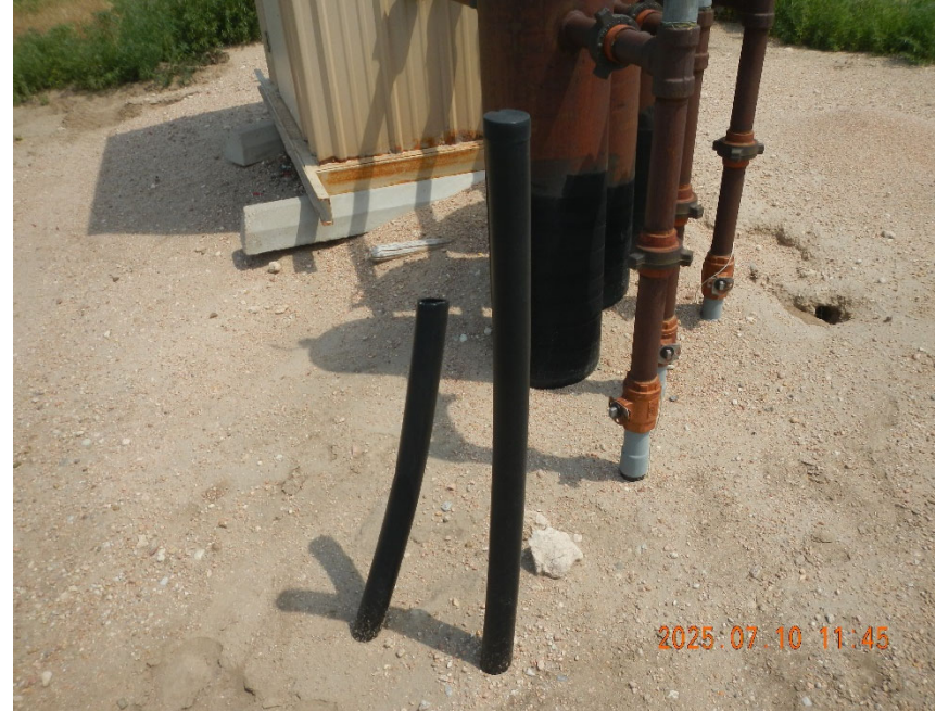
6. View of open ended stubbed up poly line at gathering location.
