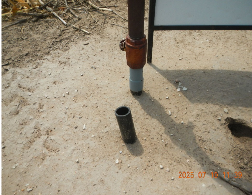
3. View of open ended stubbed up poly line at wellhead.
