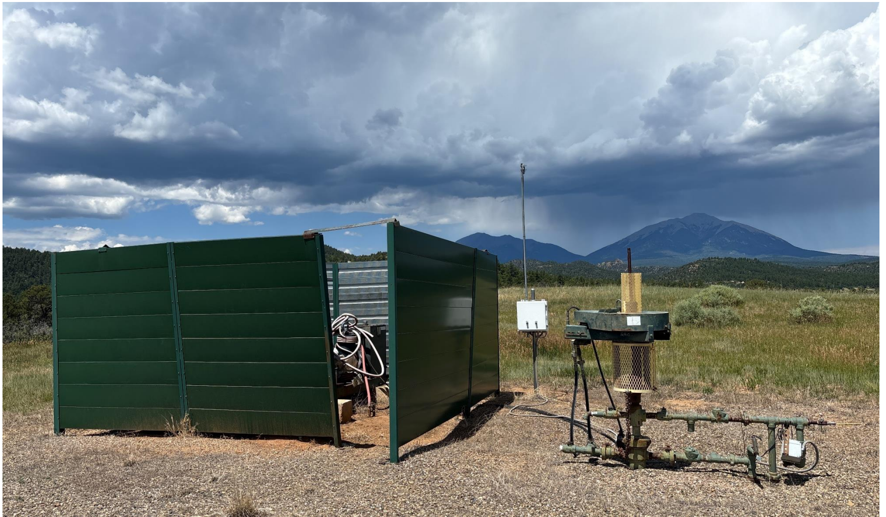
PHOTO 3: WELLHEAD AND EQUIPMENT.
