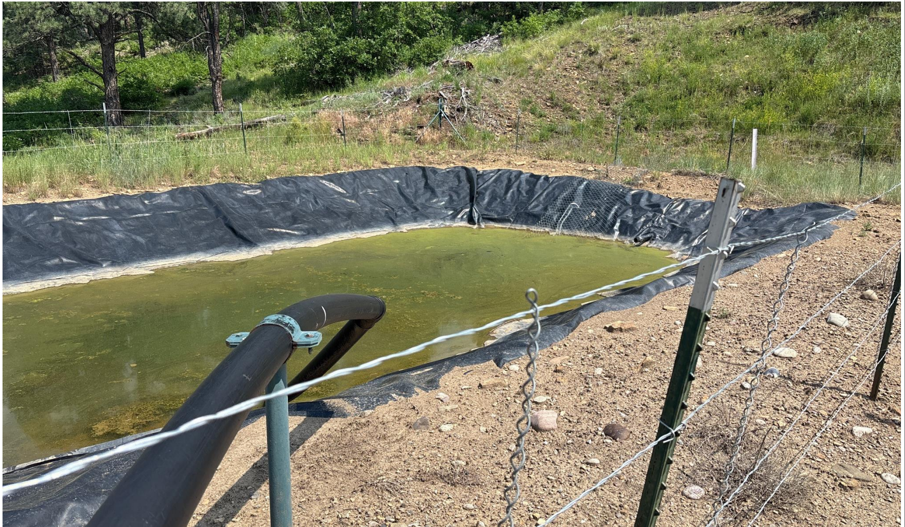
PHOTO 4: PRODUCED WATER PIT.
