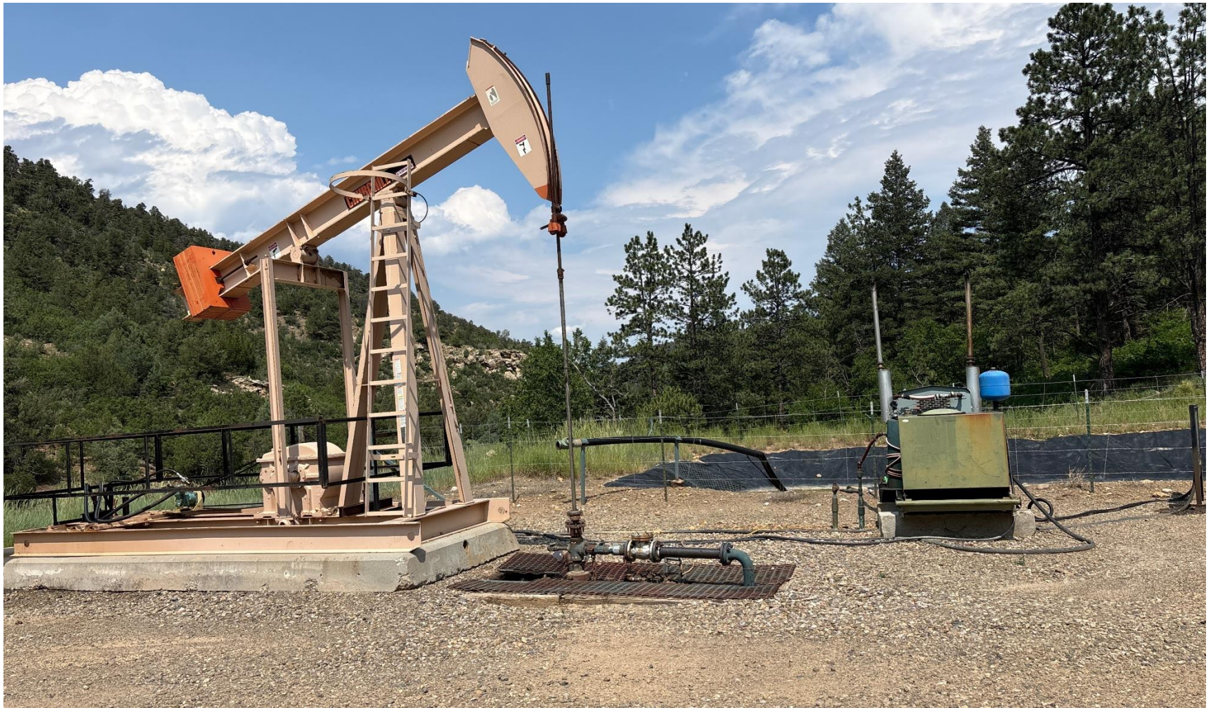
PHOTO 3: WELLHEAD AND EQUIPMENT.
