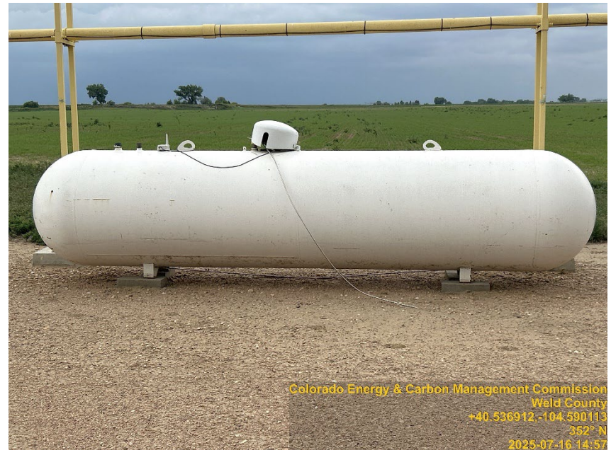
Photo #6 Faulkner 30-44 Battery site Inactive | Shut-down Propane tank placarding: Needs applied
