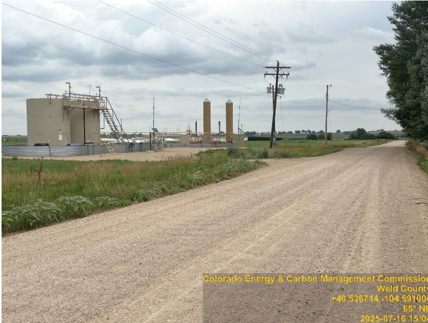
Photo #4 Faulkner 30-44 Battery site Inactive | Shut-down Wellsite(s), Battery entrance
