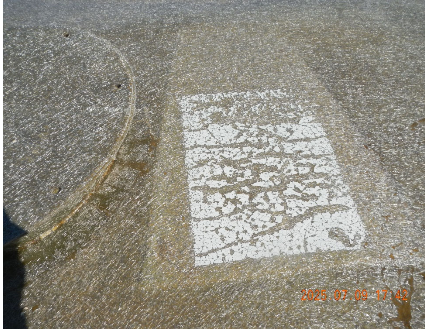
5. Produced water tank label is unreadable.
