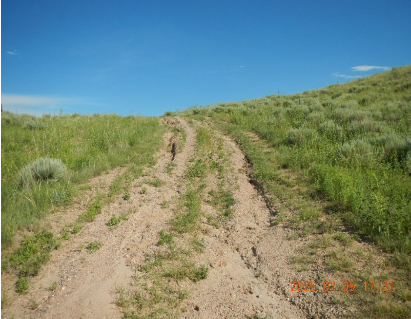
7. Erosion on access trail looking up the grade to well location.
