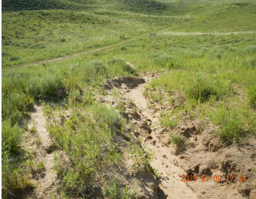
11. View of erosion channel as it continues down grade.
