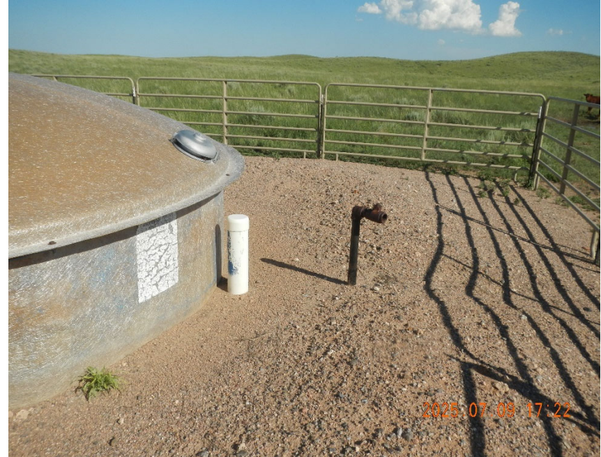
4. View of unreadable tank sign and riser at tank.wellhead.
