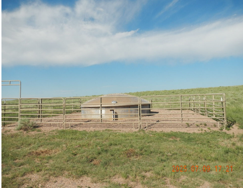
5. View of Production Tank area.
