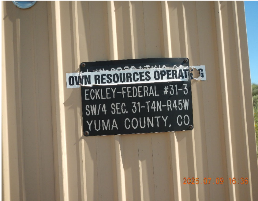
1. Lease sign at well location. Note there is no emergency contact information posted.
