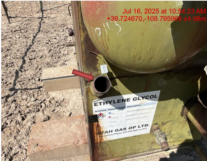
Photo # 0059 Open ended piping/wildlife hazard/available for entry by wildlife
