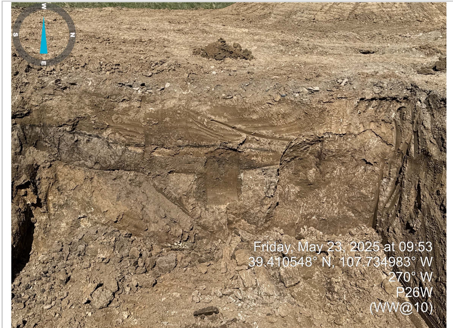
20250523-P26W-(WW)@10: View West
