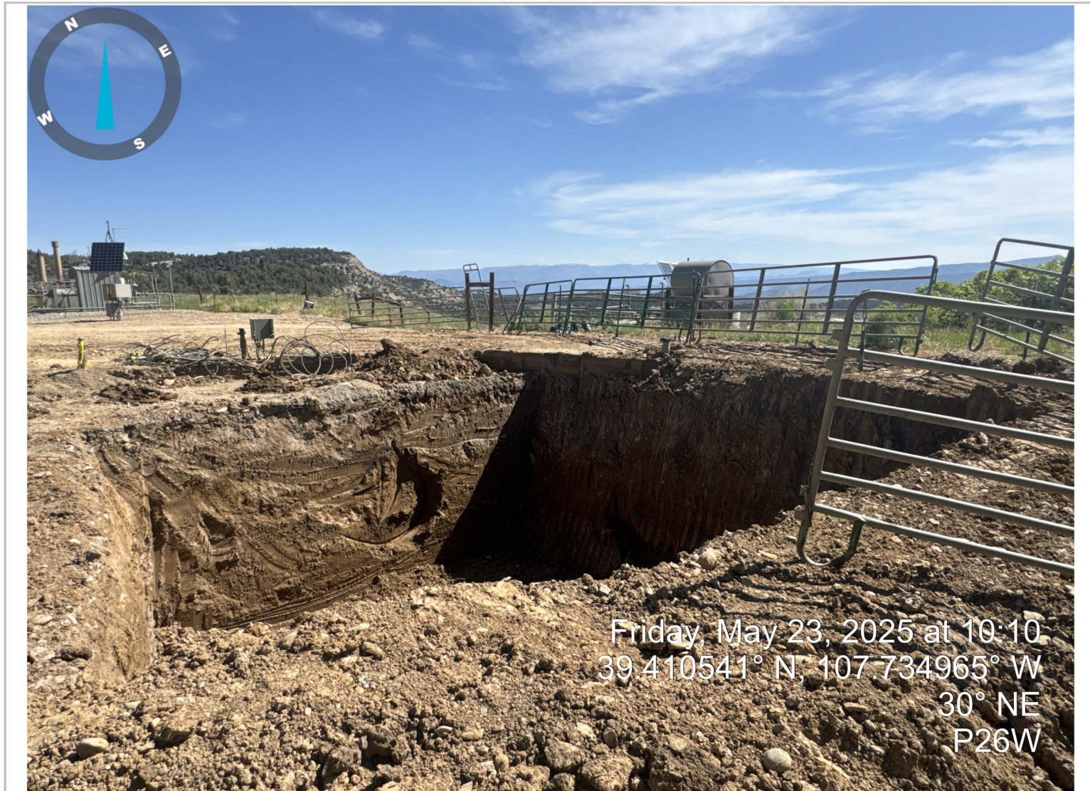
Excavation 05/23/2025: View Northeast
