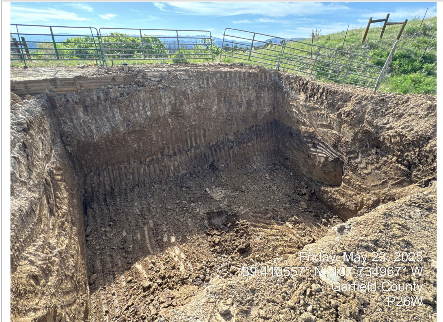
Excavation 05/23/2025: View East
