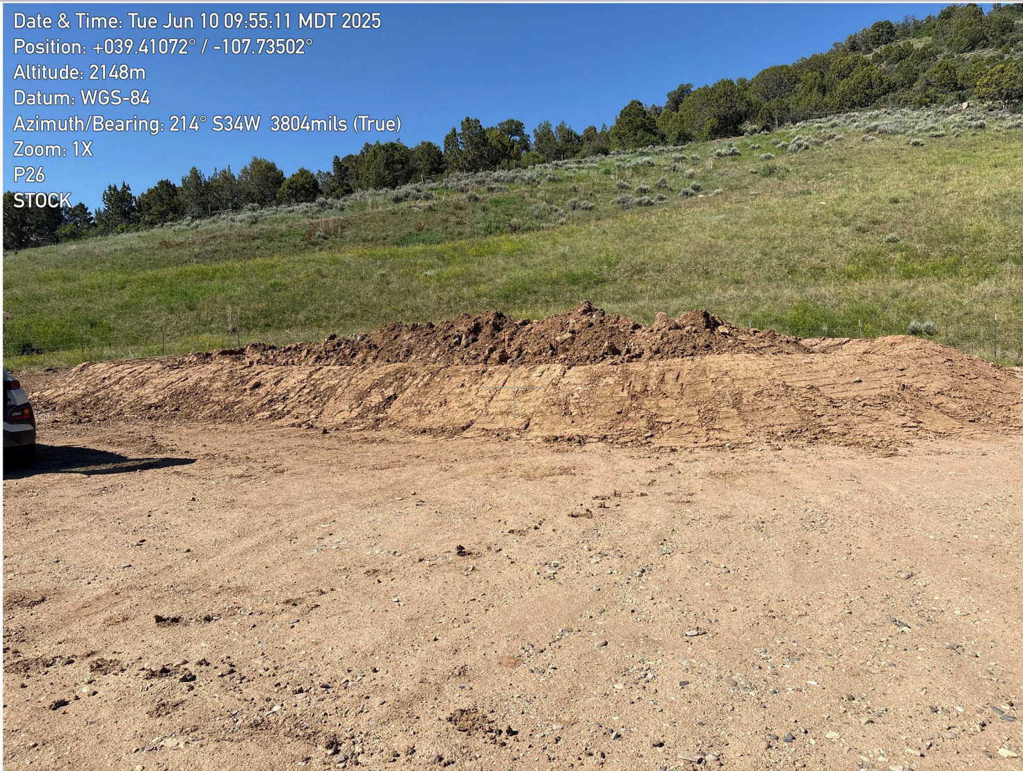
Stockpile 06/10/2025: View Southwest
