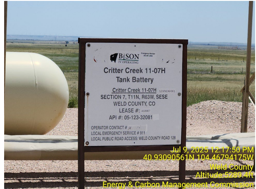
Photo 6 – Tank Battery Sign
