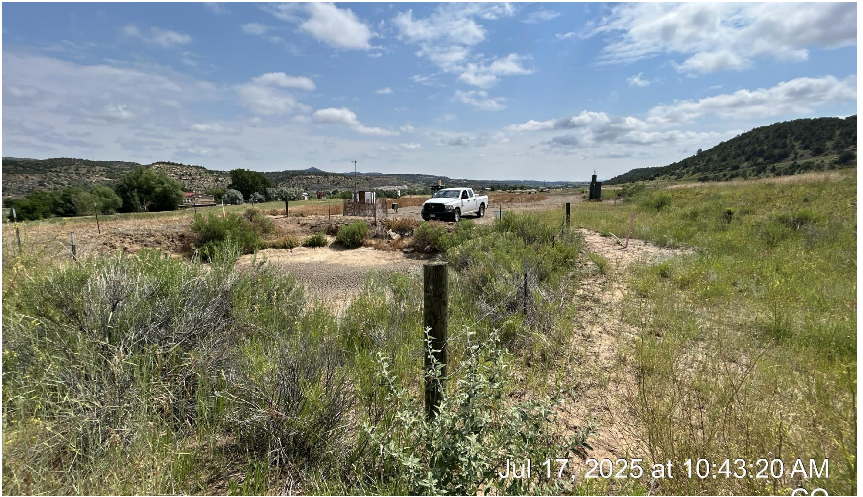
PHOTO 3: Weeds in pit & inside deadmen
