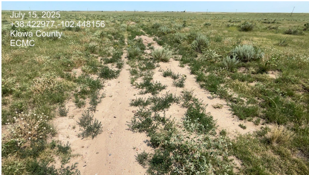
Photo 1. Facing north along the former access road. There are areas of the road that are bare of vegetation and areas that were not recontoured.
