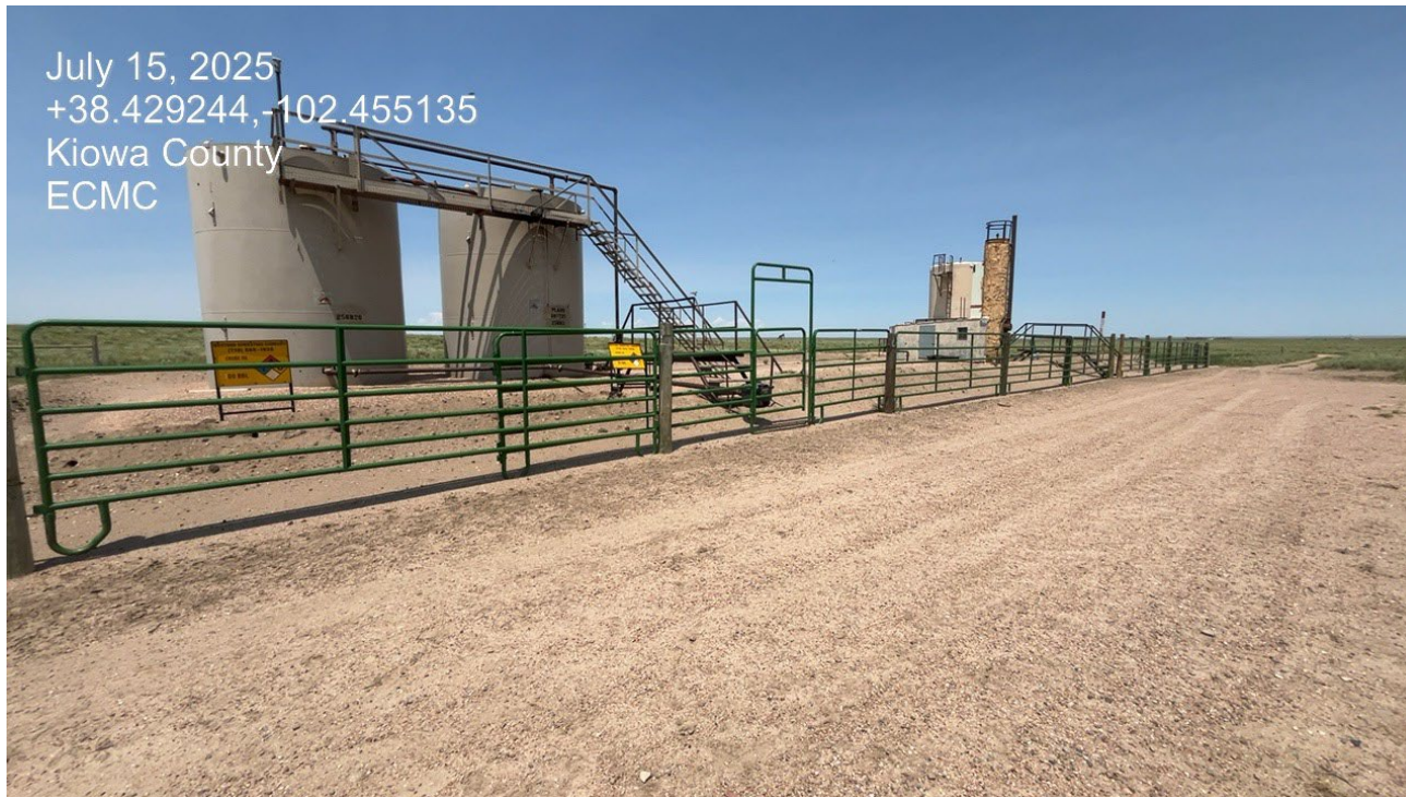
Photo 4. Facing northwest toward the tank battery.
