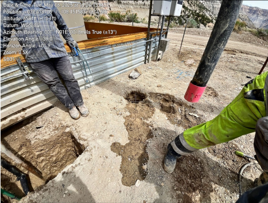
View facing north of SB01.
