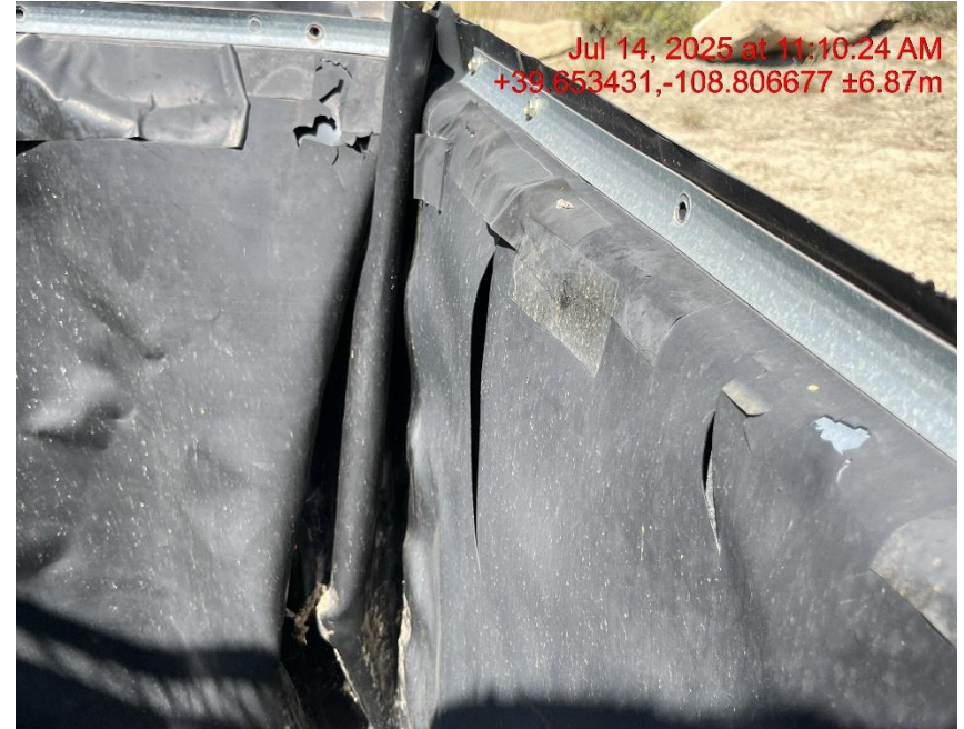
Photo # 9782 Multiple holes/tears in secondary containment liner/liner needs maintenance/liner lacks integrity
