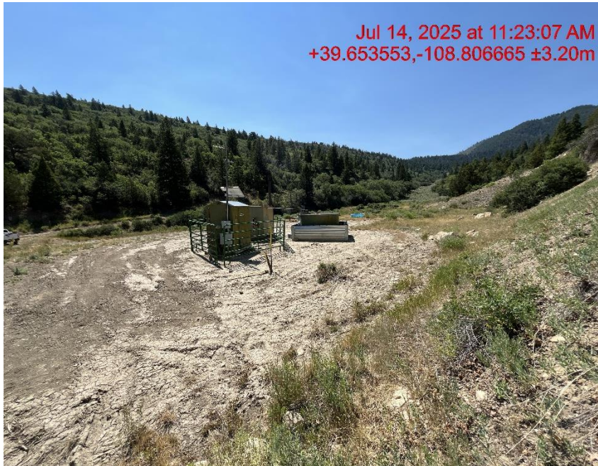
Photo # 9798 NW corner of location
