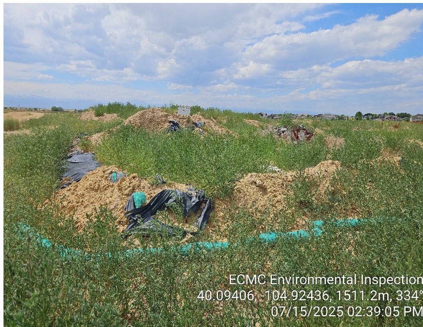
Photo 7 – Contaminated soil stockpile. Weeds/torn liner.
