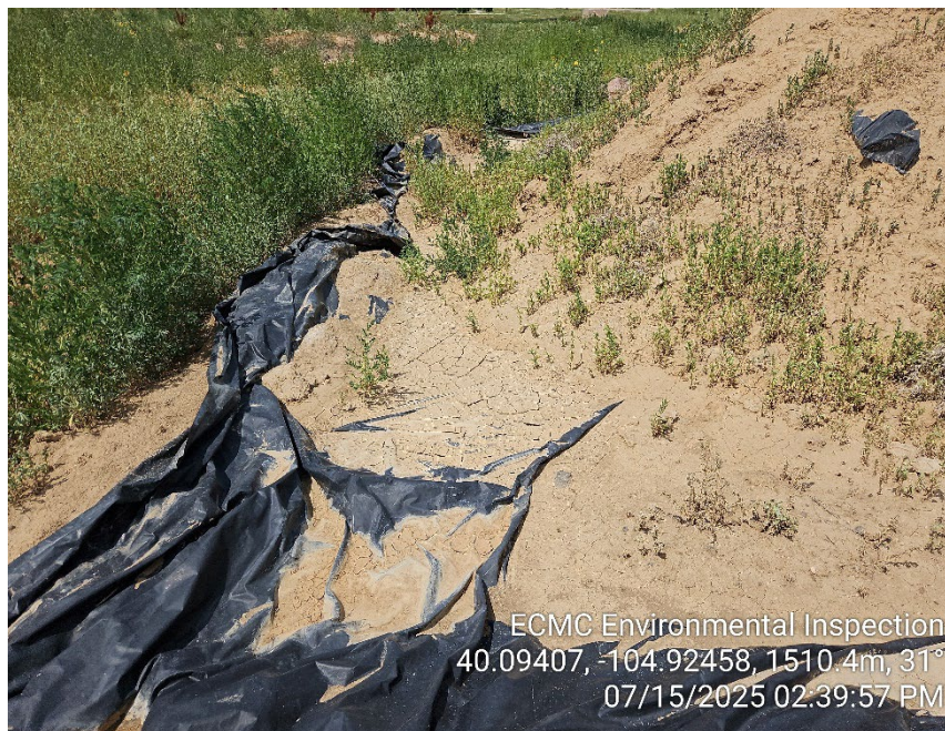
Photo 9 – Contaminated soil stockpile. Soil stockpile overflowing berms. Weeds.
