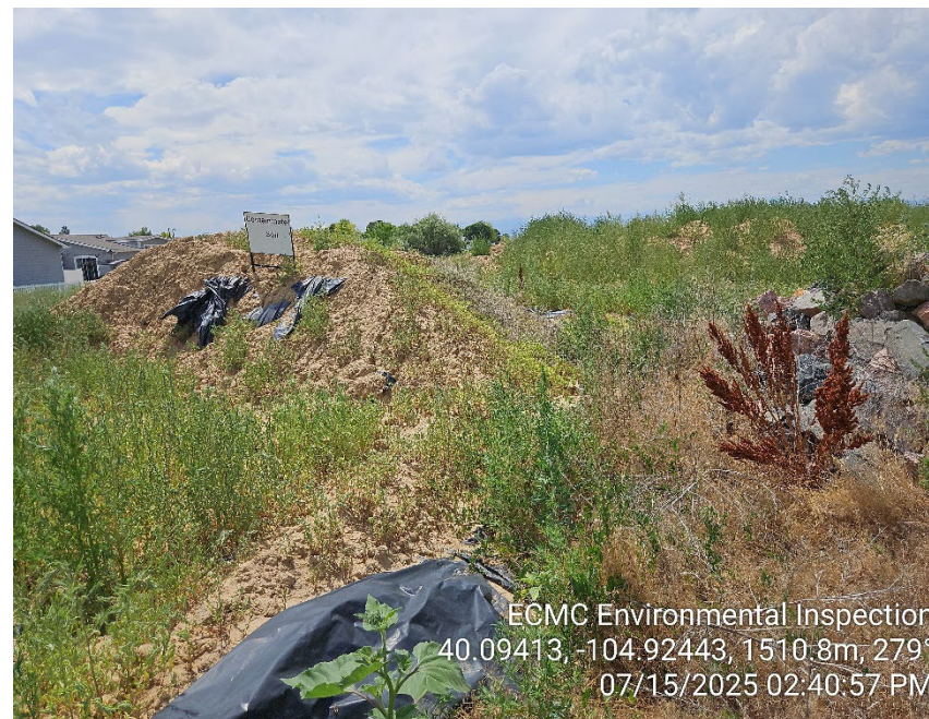
Photo 10 - Contaminated soil stockpile. Soil stockpile overflowing berms. Weeds.
