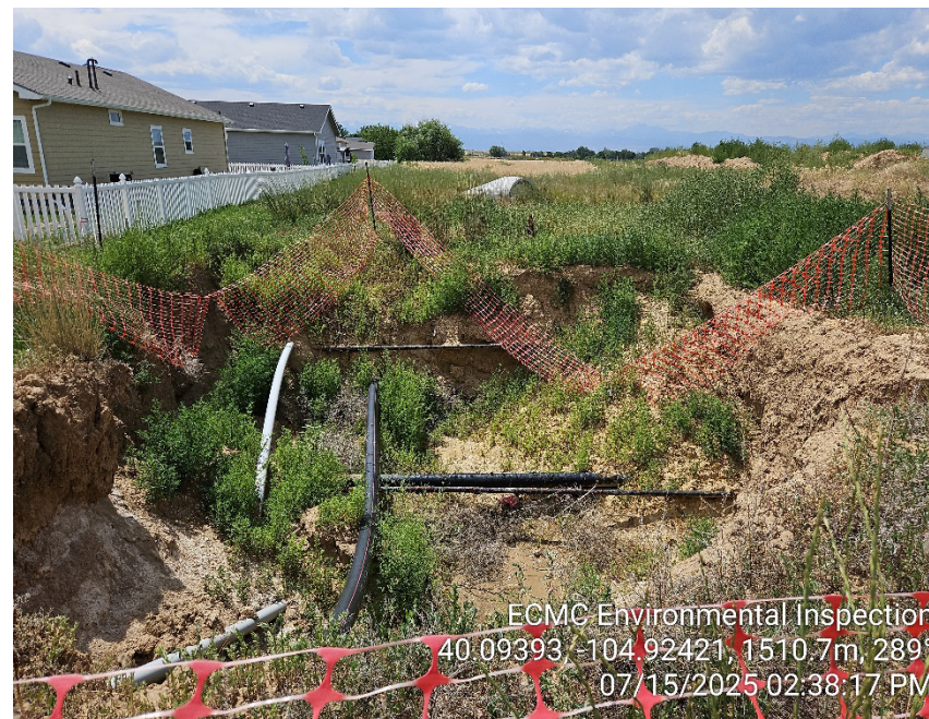
Photo 2 - Open excavation. Downed fencing/weeds.
