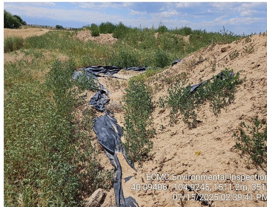
Photo 8 - Contaminated soil stockpile. Soil stockpile overflowing berms. Weeds.
