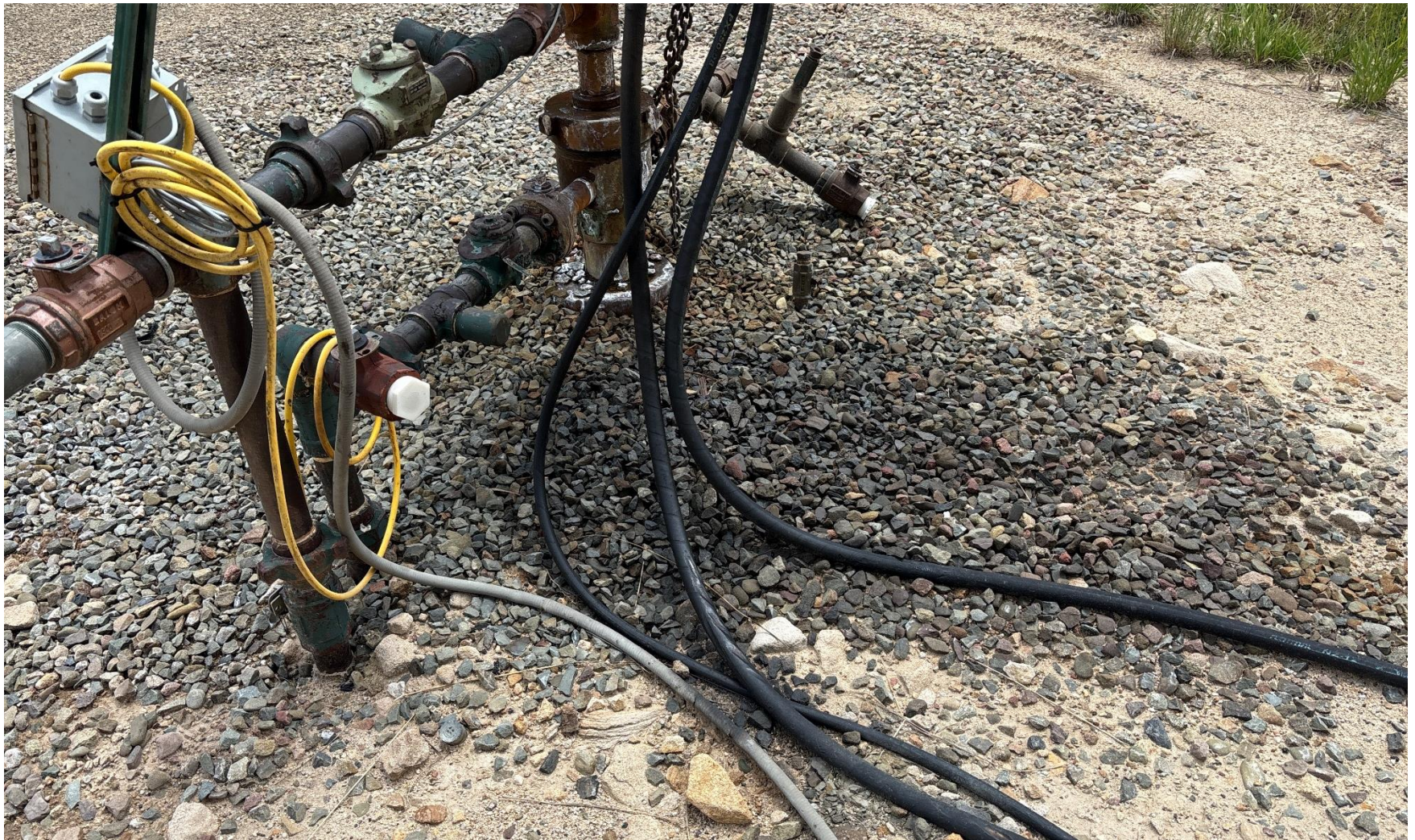
PHOTO 7: AREA OF IMPACTED SOIL NEAR WELLHEAD. Conduct maintenance on equipment, cleanup stained material and review self inspection processes. COMPLY WITH RULE 1002,(2).D. CA DATE 7-25-2025.
