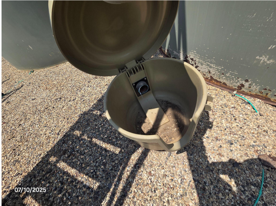
Photo 5: Photos taken from the battery facility. Photos show lines at tanks missing cap/plug.
