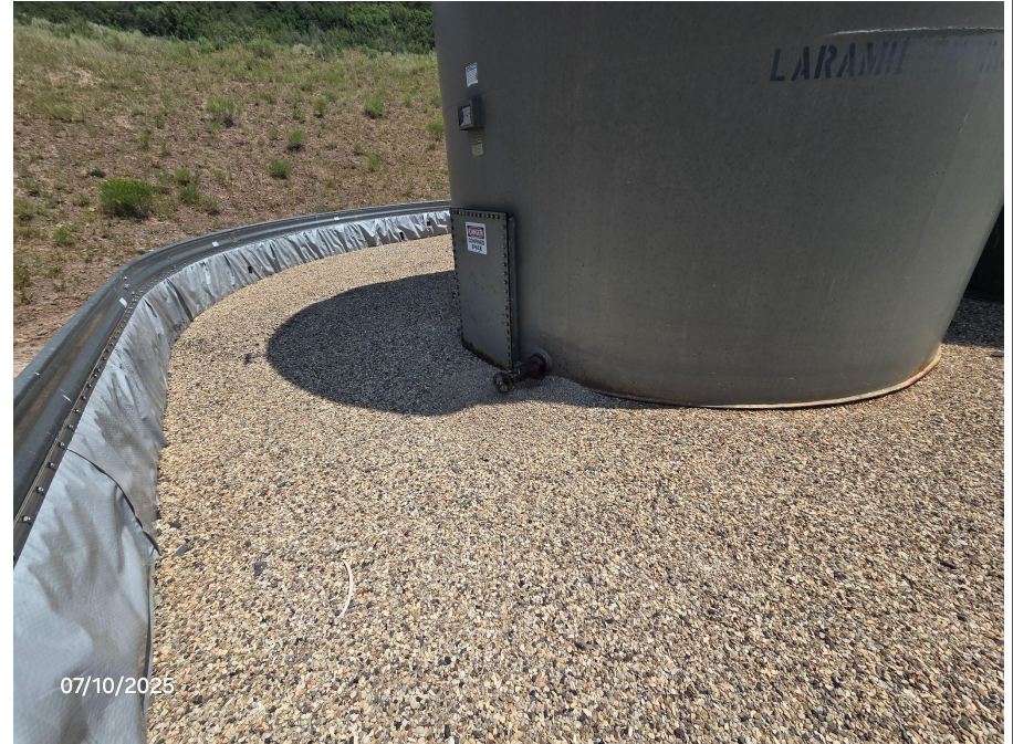
Photo 5: Photos taken from the battery facility. Photos show lines at tanks missing cap/plug.
