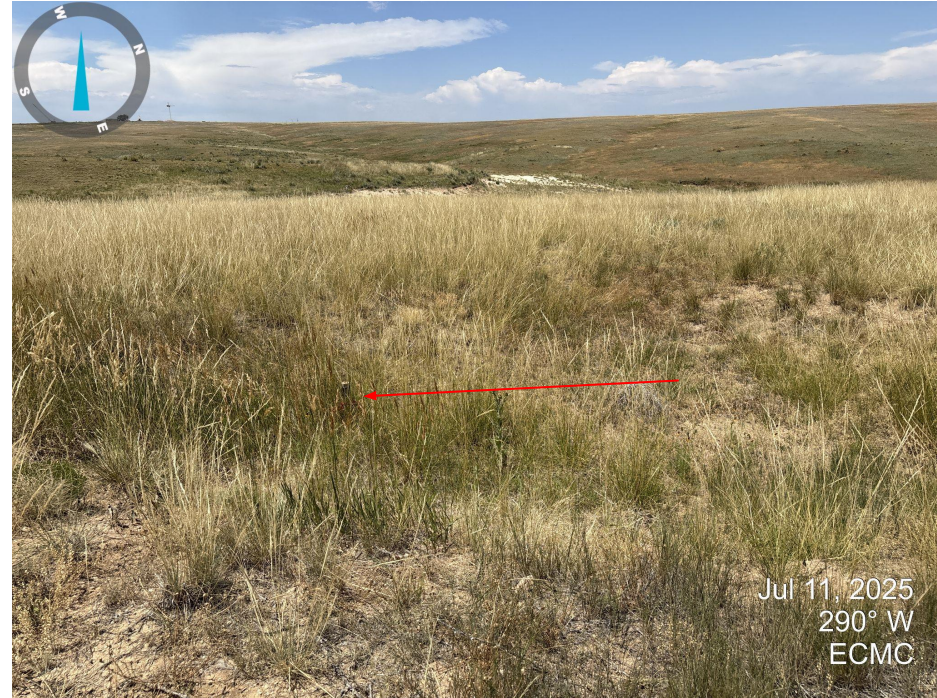
Photo 6. Looking west across the depression and exposed pipe (red arrow).
