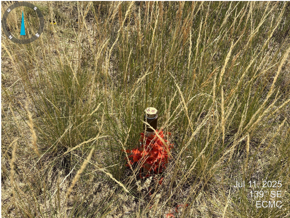
Photo 7. Picture of the exposed pipe.
