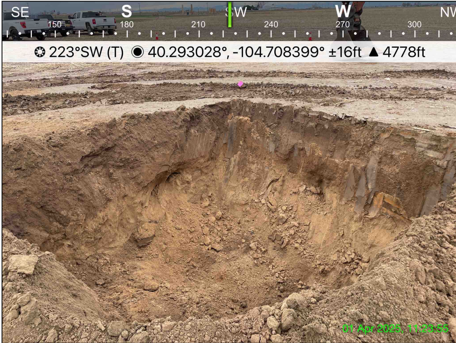
Photo 3: View of final wellhead excavation area, facing southwest.
