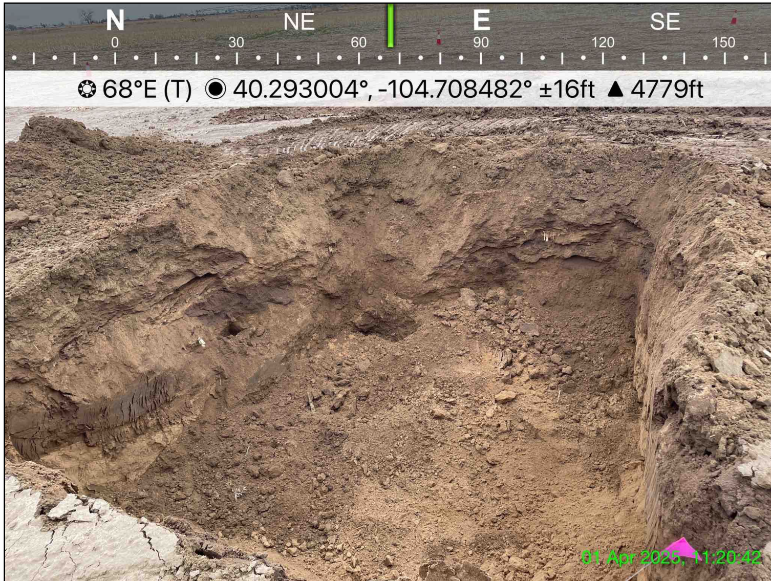
Photo 2: View of final wellhead excavation area, facing east-northeast.
